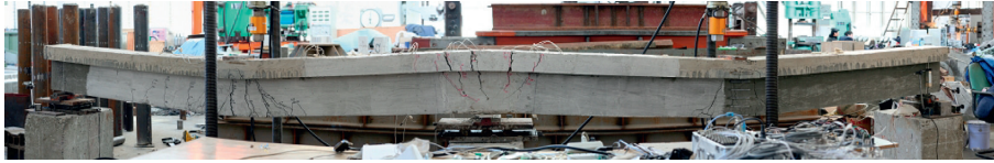
FIGURE 16: Two-span continuous composite T-shaped beams at failure.
