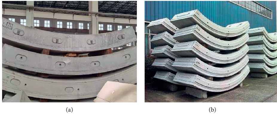
FIGURE 1: Circumferential joint. (a) Distributed mortises and tenons. (b) Full-ring mortises and tenons.
