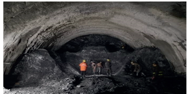
FIGURE 2: Three-bench circular excavation with reserved core soil method.
