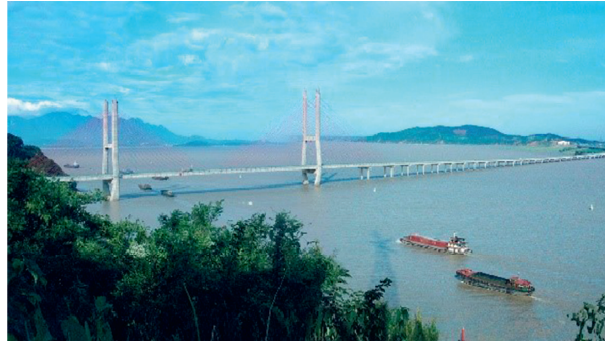
FIGURE 1: View of Poyanghu Bridge.
