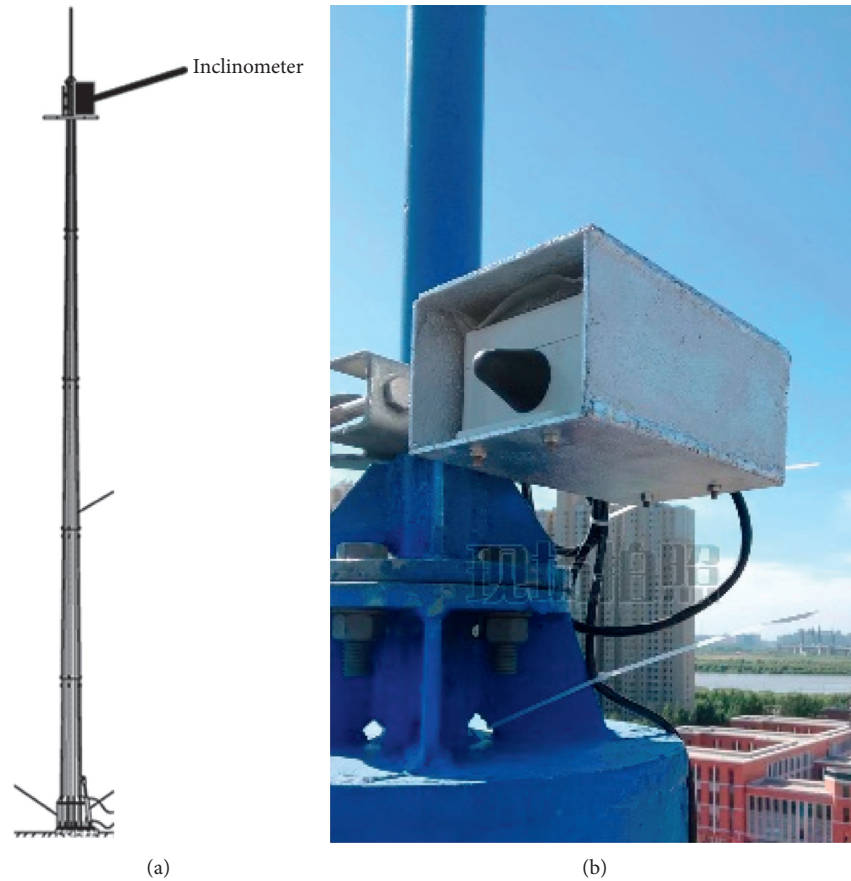
FIGURE 4: The installation of the SHM system.
