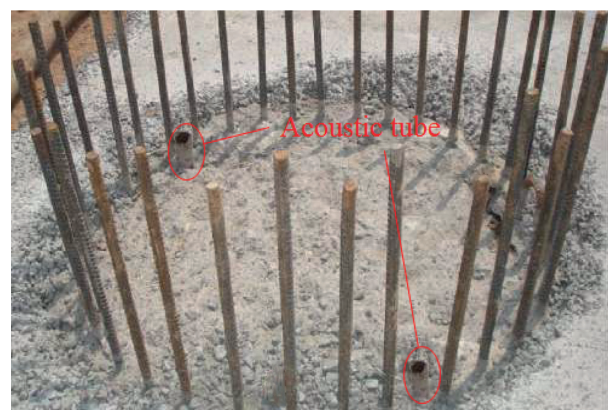
FIGURE 10: Layout of the acoustic tube.
