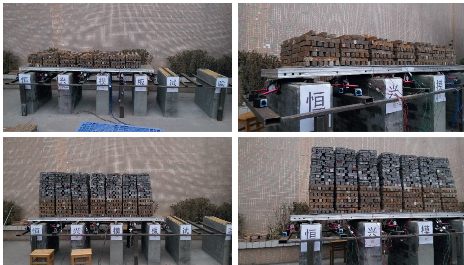
FIGURE 12: Loading process of the three-span continuous formwork.
