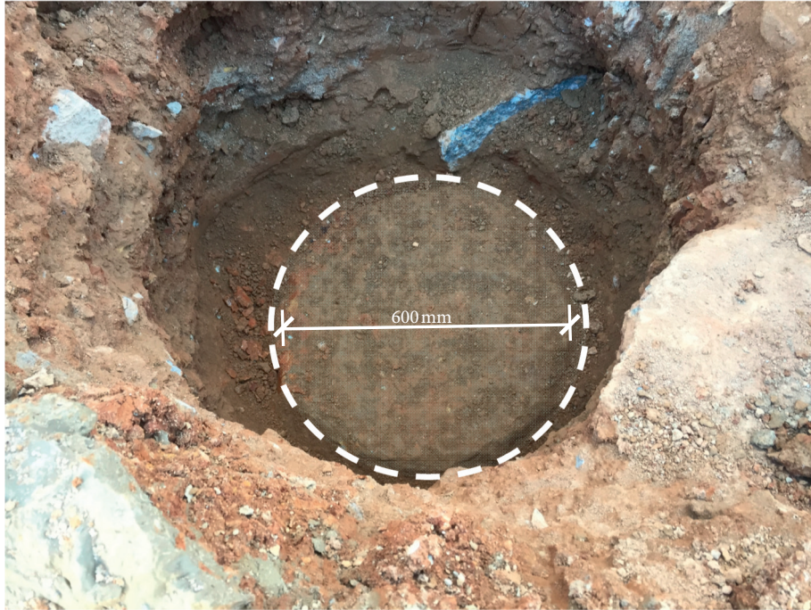
FIGURE 5: Diameter of the in situ test pile.
