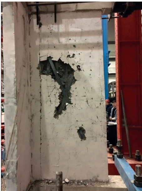
FIGURE 13: Buckling of oblique section steel.
