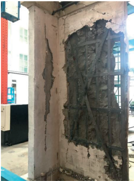
FIGURE 19: Final failure patterns.
