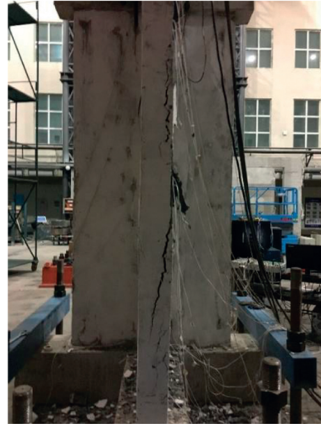
FIGURE 14: Lateral web cracks.
