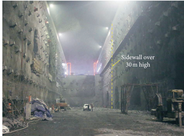
FIGURE 5: High sidewall at the underground powerhouse.
