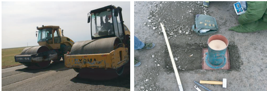
FIGURE 7: Base compacting and compaction quality detection.
