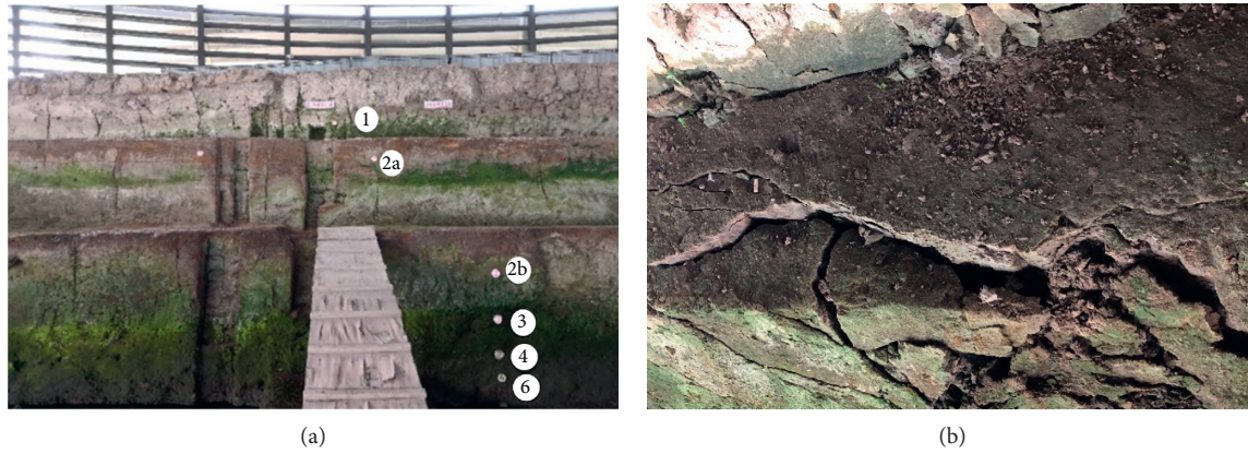
FIGURE 3: Display steps of the Tianluoshan site. (a) Display steps in the west of the site. (b) 2nd layer of soil collapse in the west of the site.
