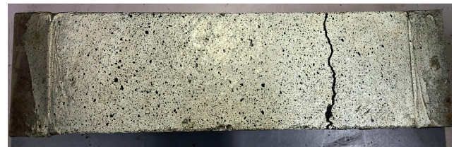
FIGURE 6: Crack patterns of RSCC-5% test specimen.
