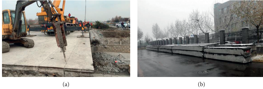
FIGURE 1: In situ construction: (a) demolition; (b) storage.
