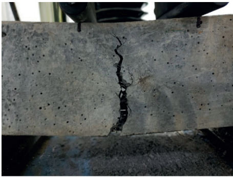
FIGURE 10: Failure condition of flexural specimens.
