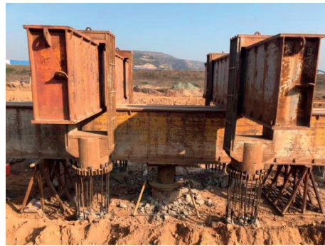
FIGURE 1: Static load test of the pile.
