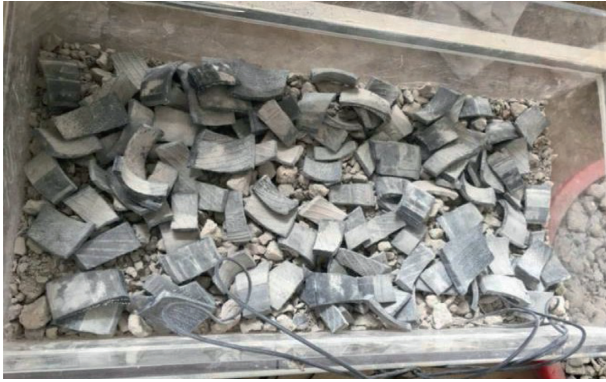
FIGURE 7: Laying of tire slices.
