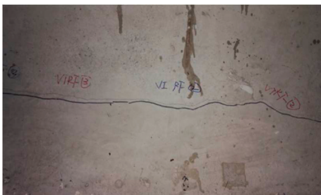
FIGURE 19: Destruction diagram of the right arch foot of the tunnel entrance section.
