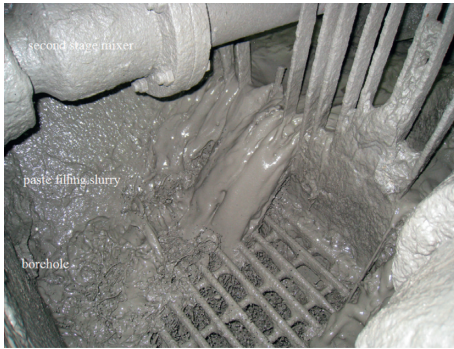
FIGURE 6: Paste filling slurry flowing into borehole.
