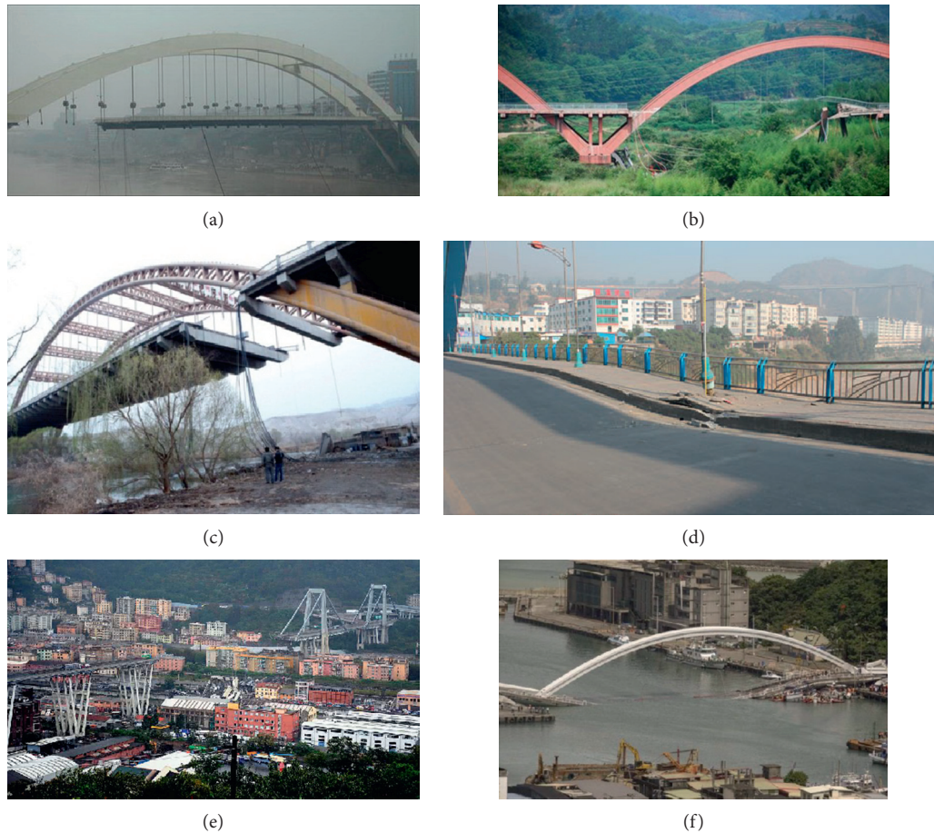
FIGURE 1: Cable breaking cases of cable bridges [1]: (a) Yibin little south gate bridge; (b) Peacock river bridge, Xinjiang; (c) Wuyishan mansion bridge, Fujian; (d) Sichuan Jinsha River Luoguo bridge; (e) Ponte Morandi bridge, Italy; (f) South Australia sea crossing bridge in Taiwan Province.
