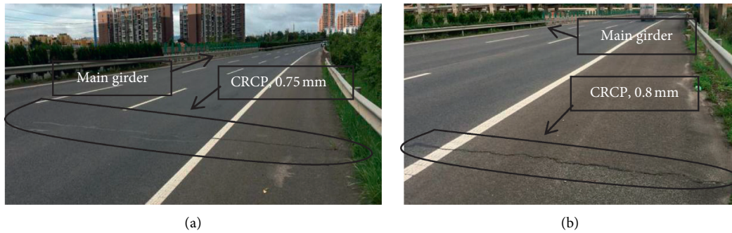
FIGURE 2: Photos of cracks in CRCP during service of fully jointless bridge: (a) Lihecun fully jointless bridge (in Feb 2019) and (b) Xinrong No.1 fully jointless bridge (in Feb 2019).
