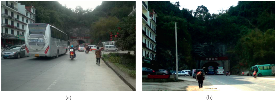
FIGURE 3: Congested road section of tunnel.
