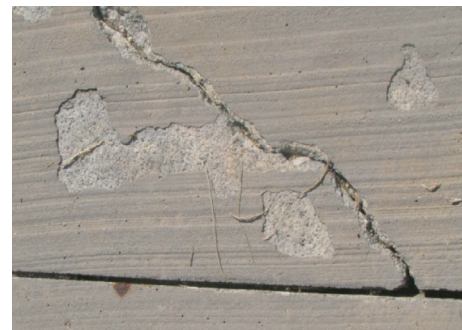
FIGURE 3: Scaling [12].
