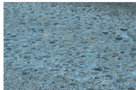
FIGURE 4: Surface polishing [12].
