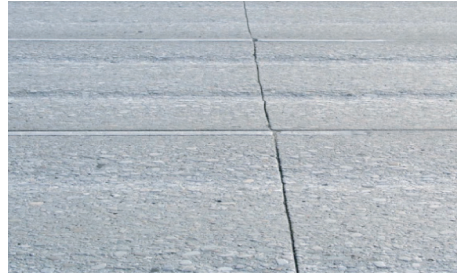
FIGURE 5: Surface wear in the wheel paths [12].
