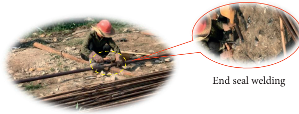
FIGURE 3: Electric welding process of steel tube.
