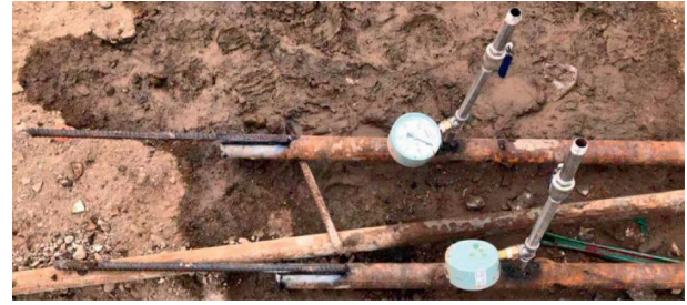
FIGURE 9: Threaded steel bar welding.
