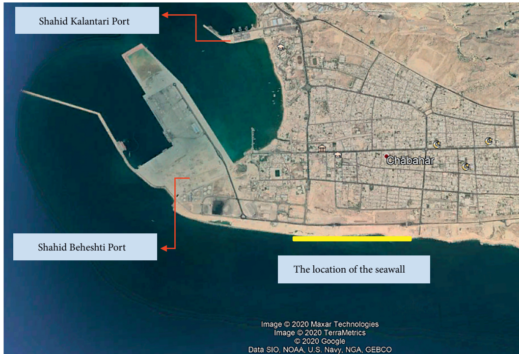
FIGURE 1: Aerial photo from Chabahar port and the location of the seawall.
