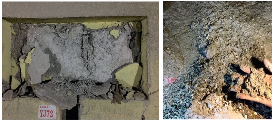
FIGURE 12: Photographs of the corroded tunnel lining concrete.
