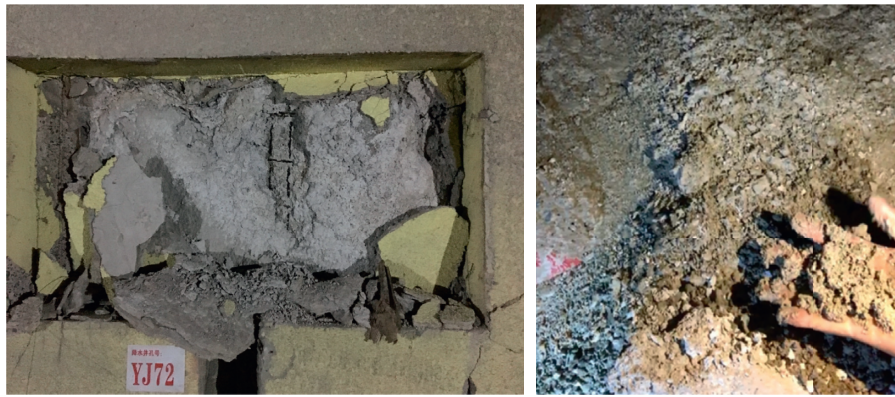
FIGURE 2: Photographs of the corroded tunnel lining concrete.
