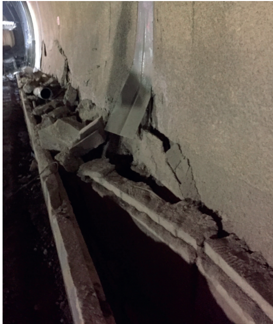
FIGURE 6: Inner wall extrusion of the cable trench.
