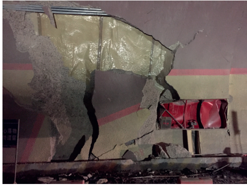
FIGURE 5: Sudden collapse of the secondary tunnel lining.
