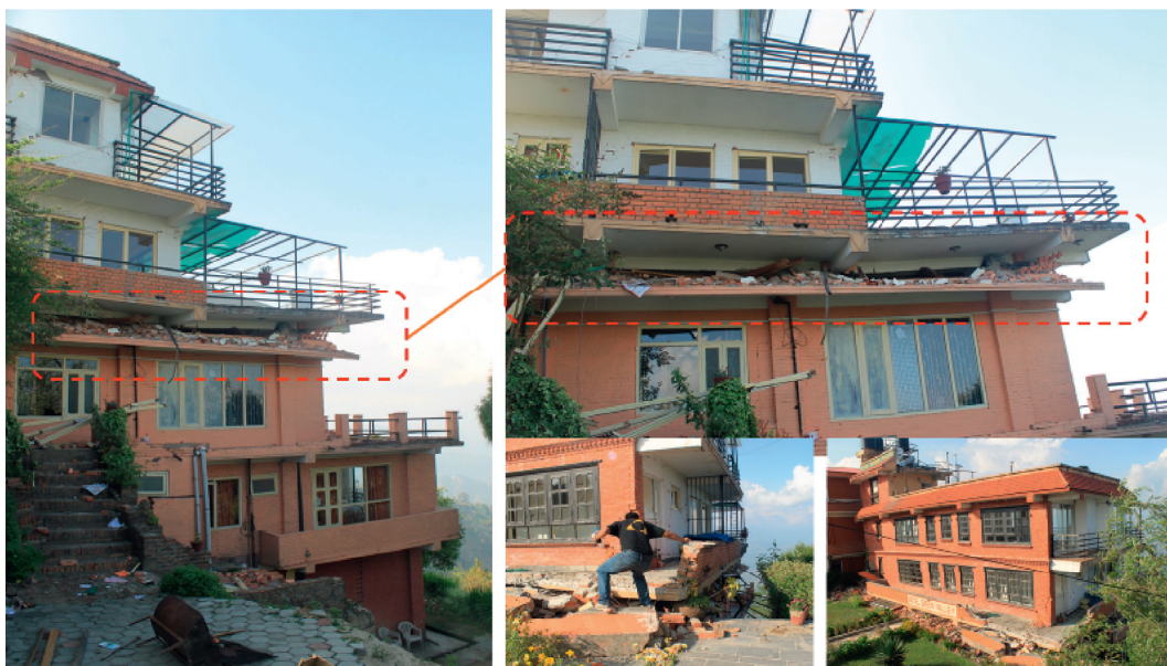
FIGURE 4: Intermediate story collapse in a modern hotel building compliant to the prevalent code at Nagarkot, Bhaktapur, Nepal.
