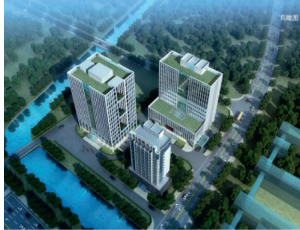
FIGURE 4: The case study project for the “CJ building.”
