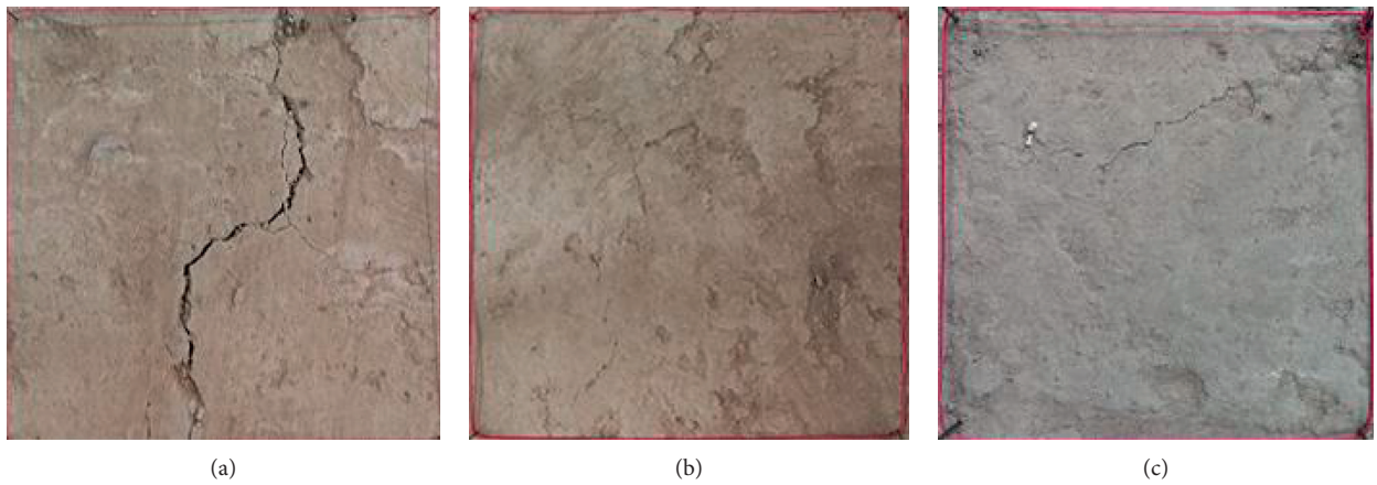
FIGURE 22: Observed cracks on the surface of base course. (a) Cemented soil. (b) Solidified soil. (c) Fiber-reinforced soil.
