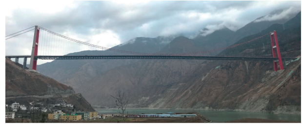
FIGURE 1: View of the Dadu river Xingkang bridge.
