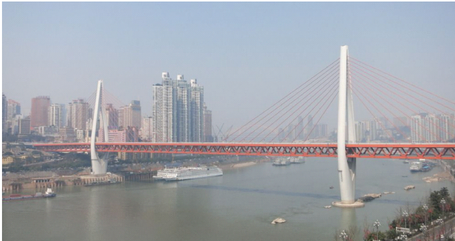
FIGURE 1: A double-pylon cable-stayed bridge with a single-cable plane and steel truss girder.
