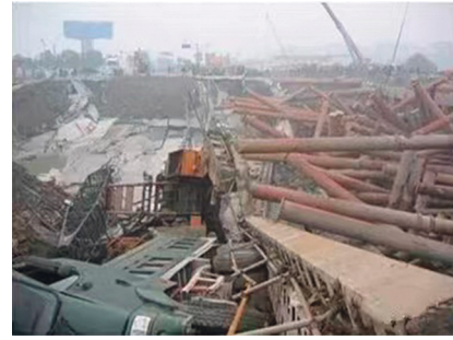
FIGURE 1: Foundation pit collapse.
