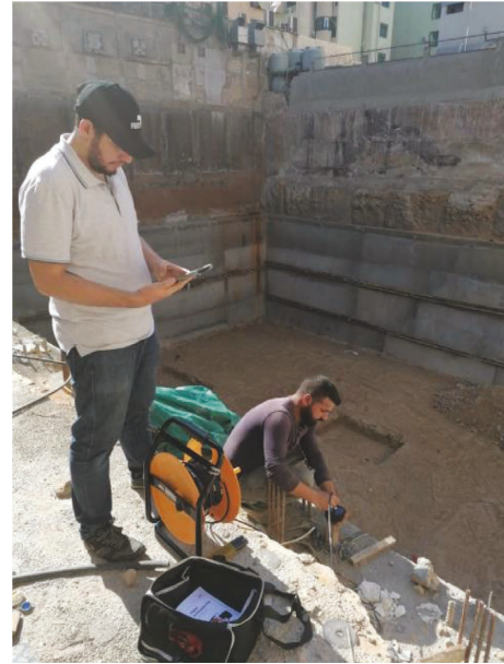
FIGURE 8: Taking inclinometer readings on-site.
