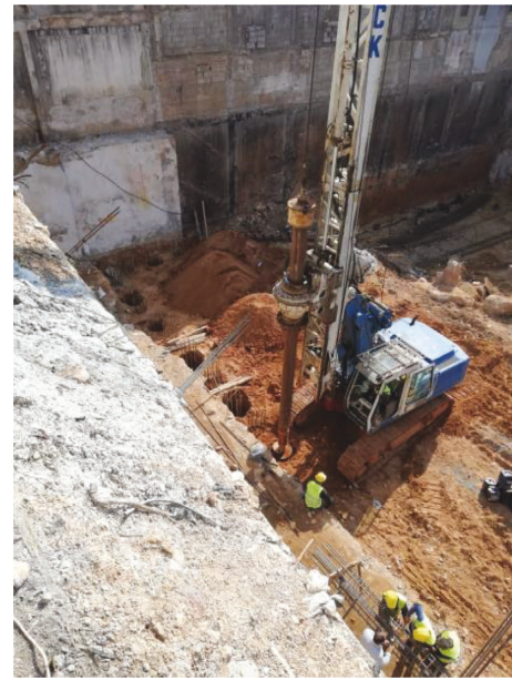
FIGURE 5: Pile hole drilling.
