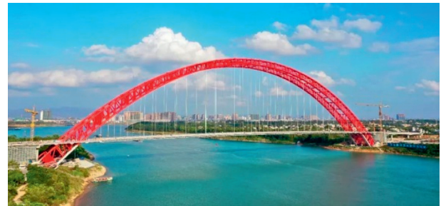
FIGURE 2: Third Pingnan Bridge.
