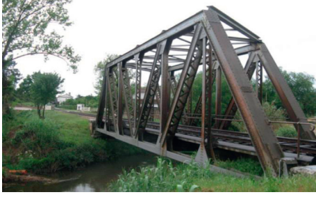
FIGURE 3: Óbidos bridge view.
