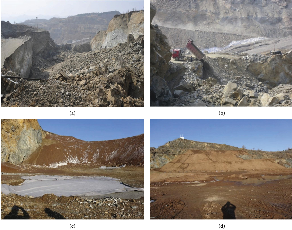
FIGURE 5: Cover of surface subsidence pit. (a) Surface subsidence pit. (b) Filling process. (c) Covering process. (d) Covering process.
