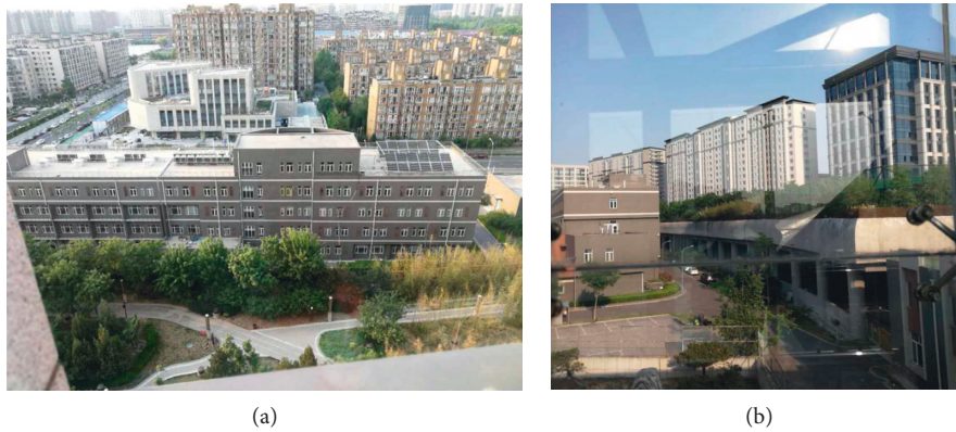
FIGURE 2: The real photos for (a) view 1: looking down angle at 15th floor and (b) view 2: looking up angle at east side.
