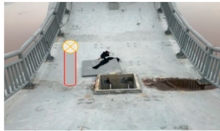
FIGURE 16: Photograph of the GNSS measuring point of the bridge tower.
