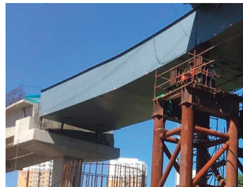
FIGURE 6: Temporary steel pier under cantilever end of the steel box girder.
