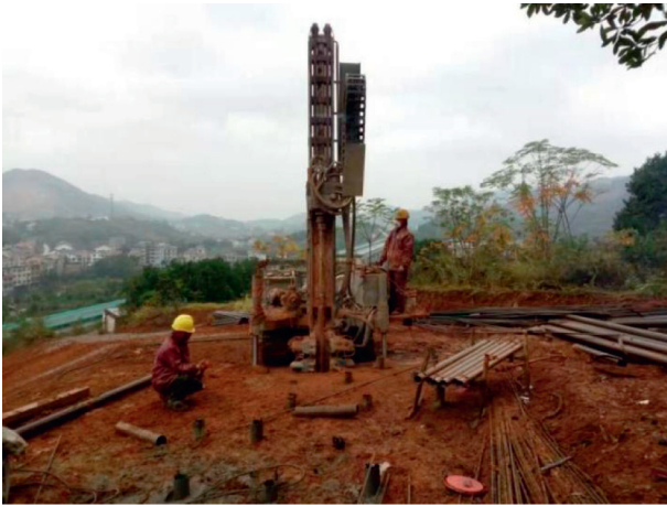
FIGURE 1: Construction process of micropiles' reinforced slope (Hunan Lou-Di, China).
