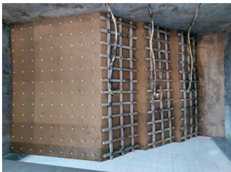
FIGURE 6: Arrangement of slope displacement monitoring points.
