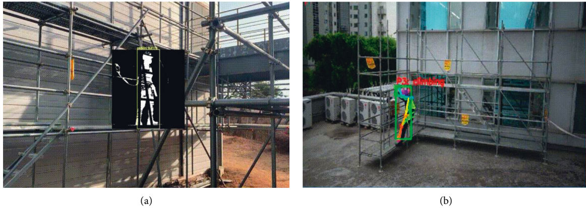
FIGURE 4: Worker detection at the sample site. (a) Worker with the safety harness and hook. (b) Climbing worker on the system scaffolding.
