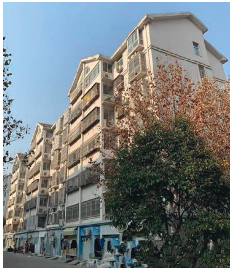
FIGURE 2: The appearance of a masonry structure.
