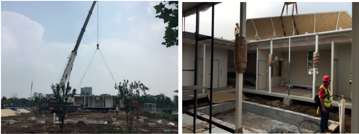
FIGURE 16: Building layout and container hoisting and splicing.
