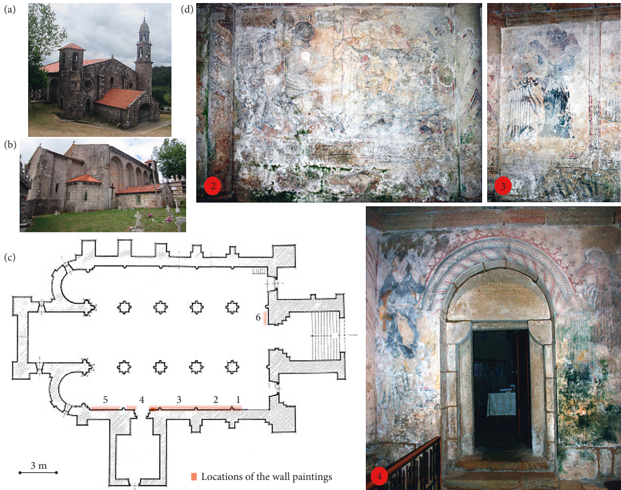
FIGURE 9: General view of the San Julián de Moraime Church (a), northern wall (b), plant view of the interior and locations of the wall paintings (c), and some of the paintings showing deterioration (d).
