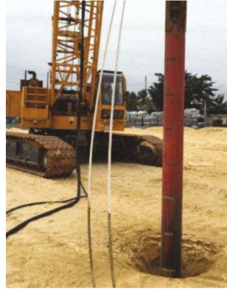
FIGURE 6: On-site vibroflotation.
