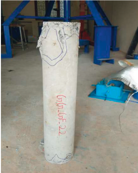
FIGURE 11: Column after being subjected to damage.
