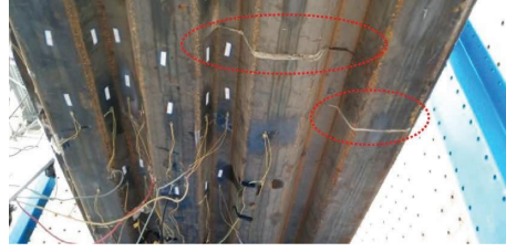
FIGURE 1: Fatigue failure of a profiled steel-concrete composite deck.
