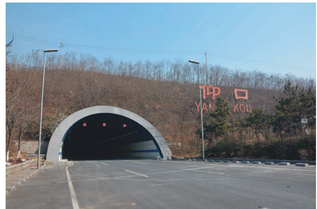
FIGURE 6: The Yangkou tunnel after rehabilitation.
