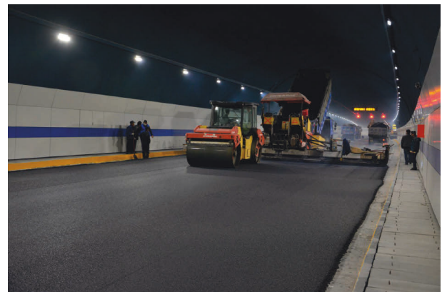
FIGURE 7: Paving new asphalt course.
