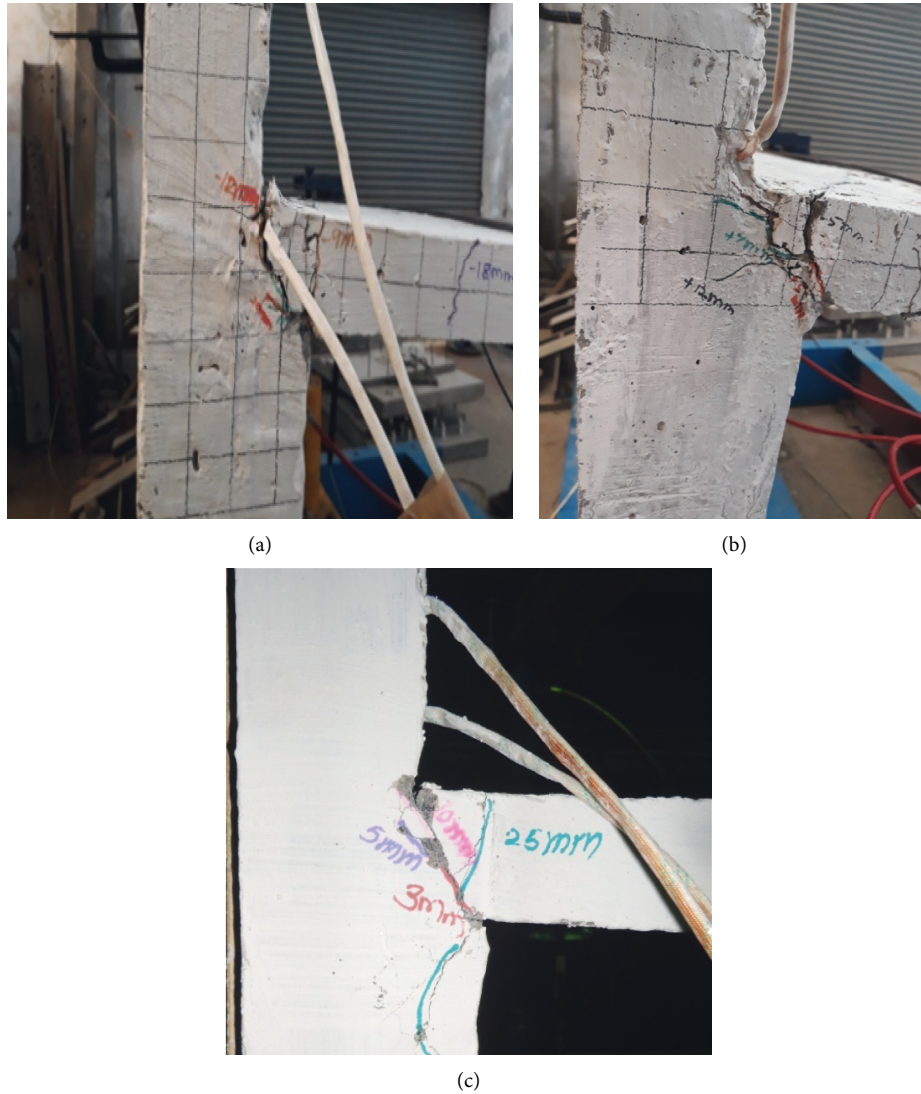
FIGURE 8: Cracking pattern of specimens in sectional view. (a) Type 1, (b) Type 2, (c) Type 3.
